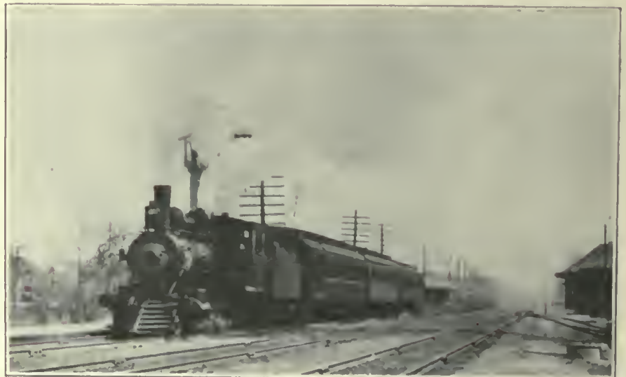
FIG. 373. SUBURBAN PASSENGER TRAINS. Suburban Train of the Chicago, Burlington & Quincy Railroad at Riverside Station. This train consists of a ten-wheel type locomotive and three coaches.
